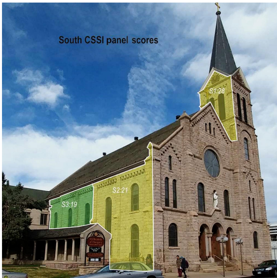
FIGURE 14.15 Saint Elizabeth's south-facing facade, displaying "Excellent" and "Good" CSSI scores. While very stable overall, the church's south aspect did have a few minor concerns, such as fissures, flaking on the underside of window arches, and very small plant growth at the facade's base.
